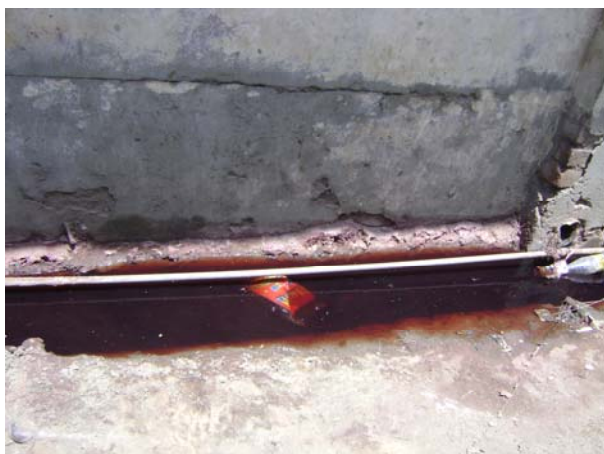
Photo 1: Open Drains Carrying Wastewater in Old Town
